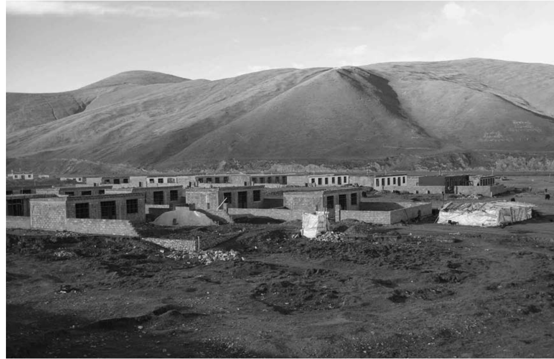
Nomad settlement camps are now under construction in many areas of eastern Tibet. This image shows a new settlement in the small town of Son mda’ (Chinese: Qingshuihe) in Kham (present-day Qinghai Province). (August 2007.) IMAGE: ICT.
