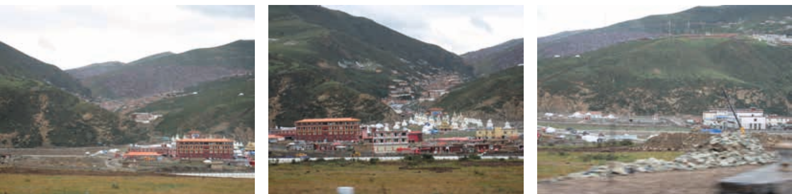
While inside the Larung Gar Buddhist Academy demolitions of monastic quarters are ongoing, outside the main entrance large-scale construction work is in progress to turn the large valley into a tourist resort with hotels and guest-houses as well as new offices and facilities for local authorities (Images: ICT).
