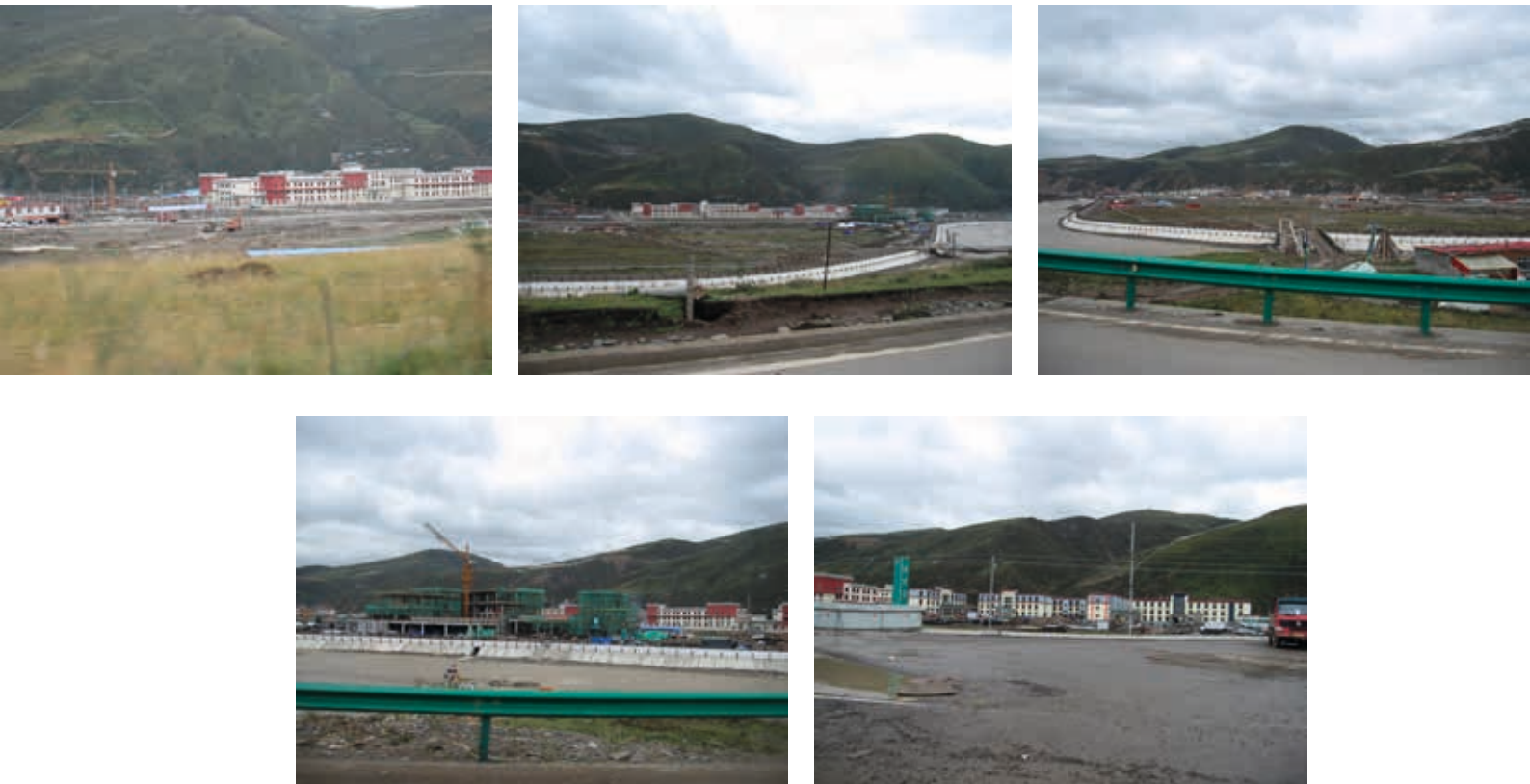
These images show ongoing construction of a large building most likely to host tourist services, guest houses, travel agencies, trekking and horse riding facilities in an attempt to boost the local economy and capitalize on the increasing cultural and spiritual attractions of Serthar among Han Chinese tourists (Images: ICT).
