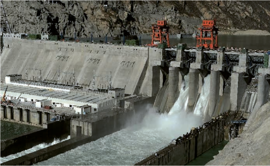
Water surges from the enormous Zangmu dam at the hydro-power station on the highest river in the world, the Yarlung Tsangpo, soon after it became operational in November, 2014. Image from the Chinese official news agency Xinhua.
